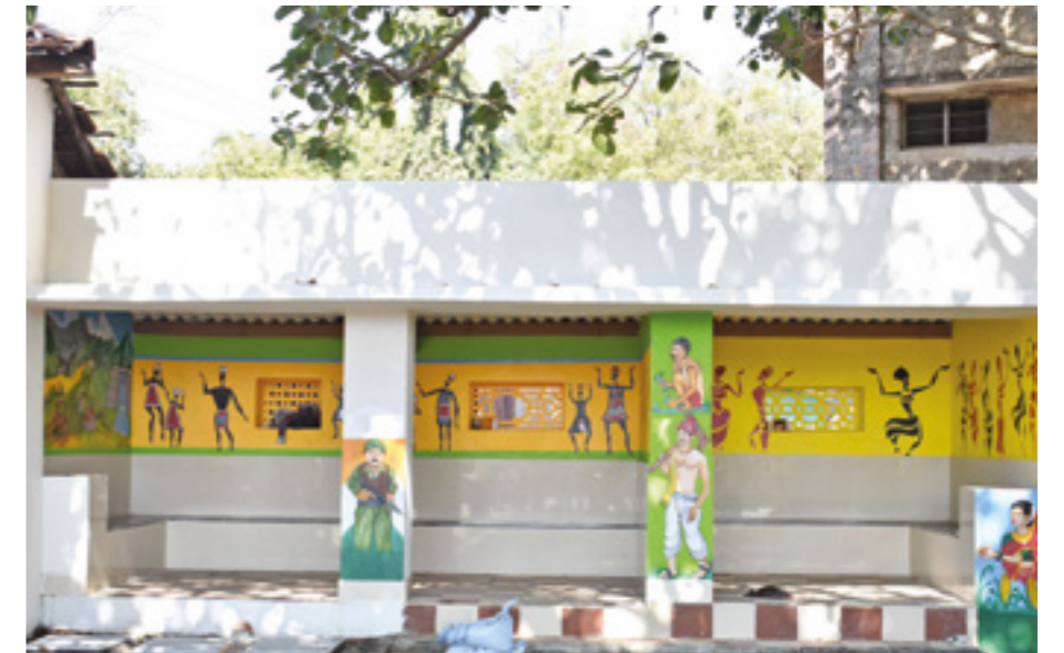
▲ Rural development - construction of bus shelter
