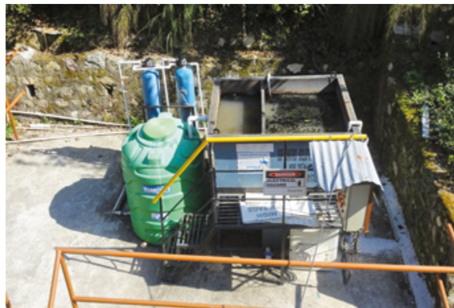
▲ Treated water is used for gardening
