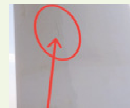
▲ Blade drone inspection
