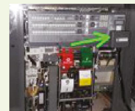
▲ WTG ACB Maintenance
